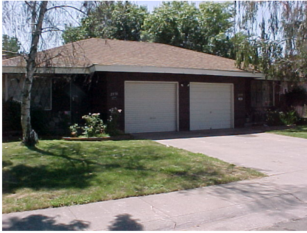
Front View of the Duplex
